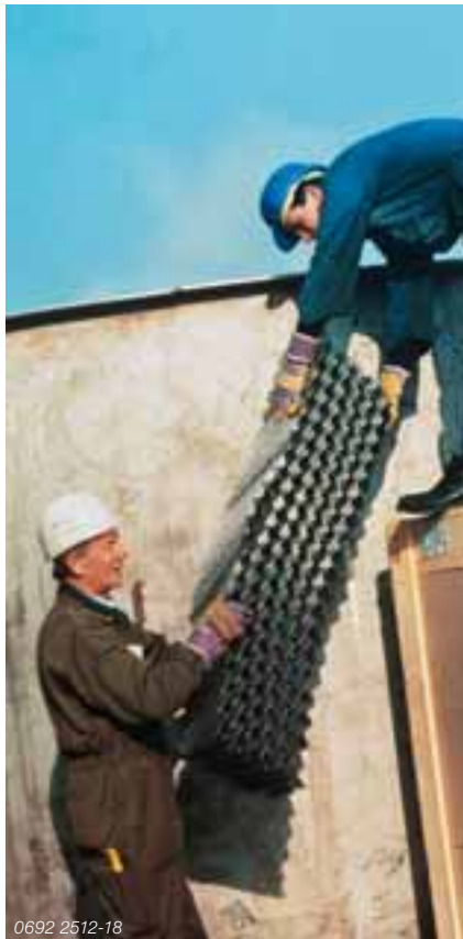
Revamping of a vacuum column with Mellapak
