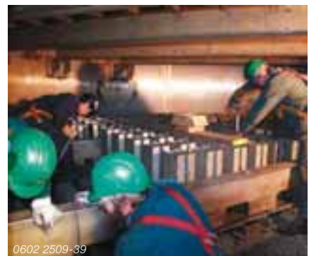
Installation of the liquid distributor
