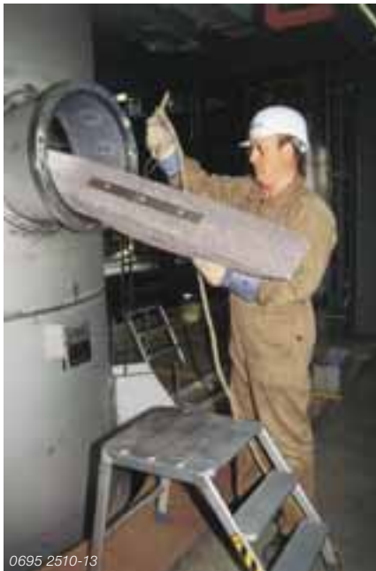
Installation of packing
