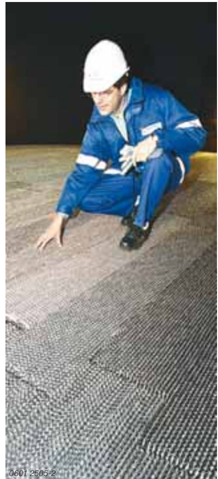
Inspecting packings after installation
