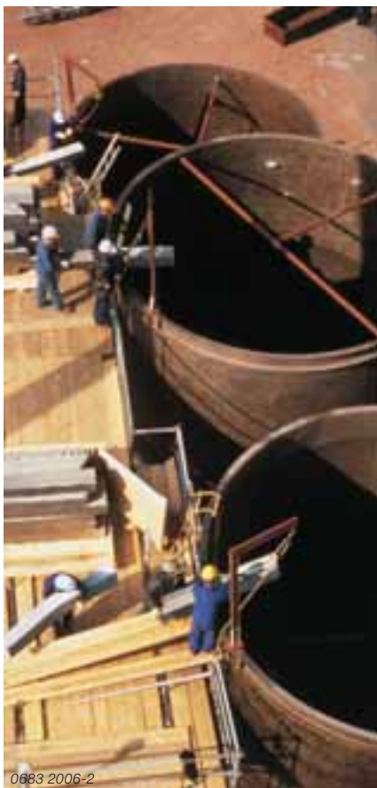
The packing is fitted inside the column sleeves at the preassembly site
